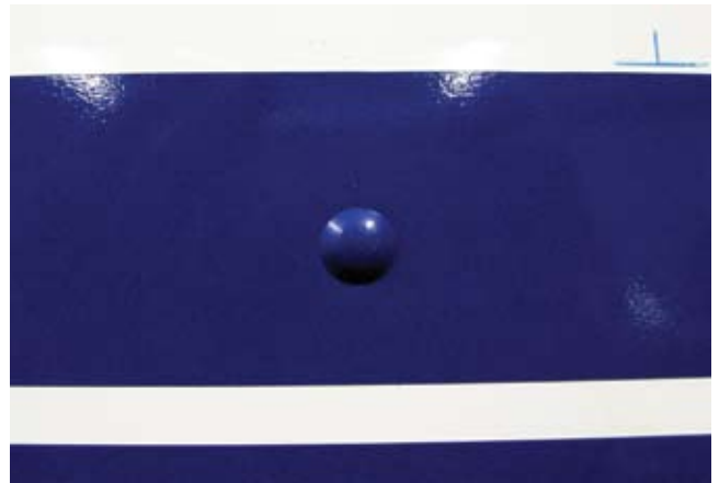
After completing the air-expulsion process with a row of rivets, heat each rivet once more to ensure they stay tight. Once air has been released, vinyl withstands substantial heat application.
