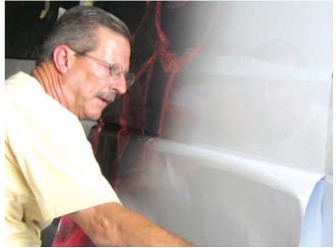
Squeegee all the way across the indentation's upper portion. To prevent bridging, bubbles and stretching, make sure it never touches the lower portion.
